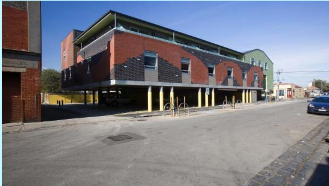
Woodstock rooming house, Balaclava (MGS Architects, photo: John Gollings)
